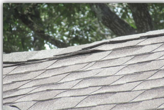
Front and Back Roof Photos
