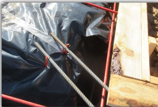
The moisture barrier is torn/incomplete in several areas and should be repaired before the concrete is poured.
