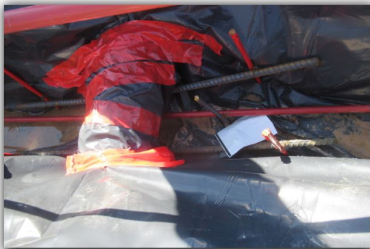
The moisture barrier is torn/incomplete in several areas and should be repaired before the concrete is poured.
