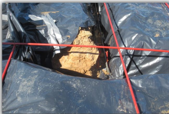
The moisture barrier is torn/incomplete in several areas and should be repaired before the concrete is poured.
